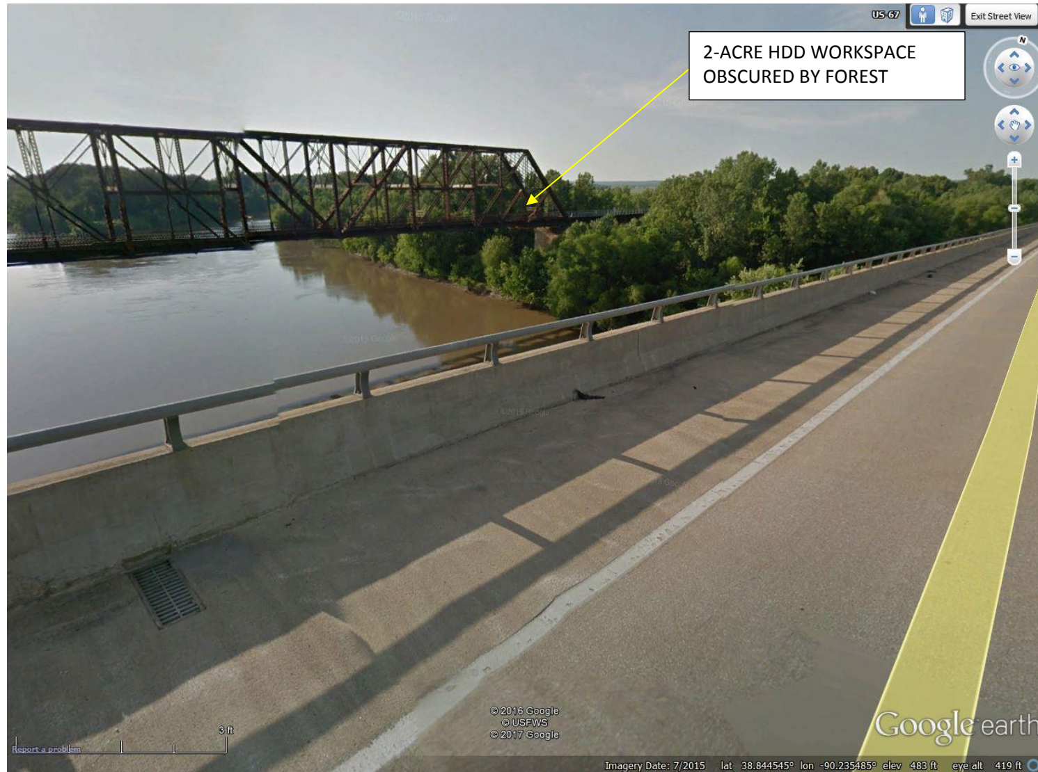
VIEWSHED 2: Missouri River Crossing From Highway 67 Bridge Facing Northwest To HDD Workspace Location.
