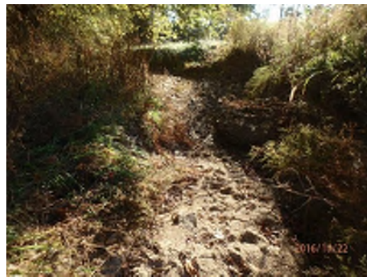
Stream SIL-TMA-048, Downstream, Facing East (10/22/16)
