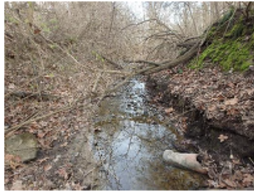
Stream SMO-JJP-015, Downstream Facing East (2/16/17)
