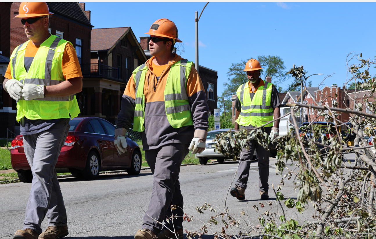
Spire crews led the effort to secure neighborhoods, identify leaks and make repairs
